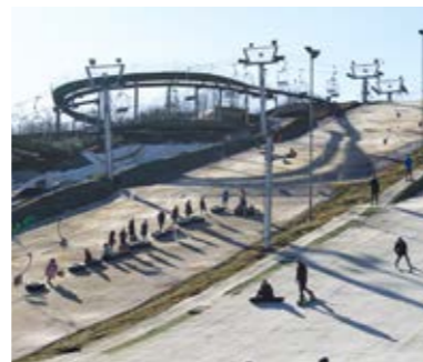
BRACKNELL SKI SLOPE
